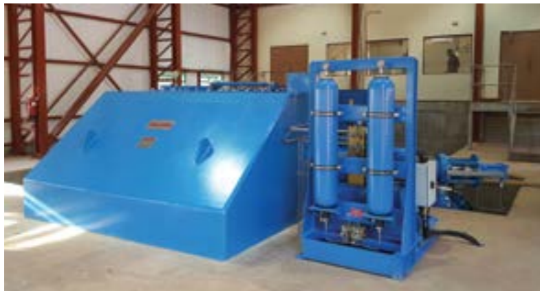
Above: 2.2MW Turgo installed 2017, Zimbabwe
