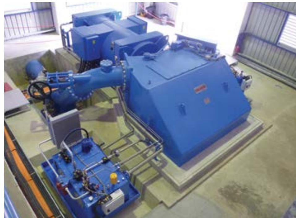
Above: 2.2MW Turgo installed 2017, Zimbabwe
