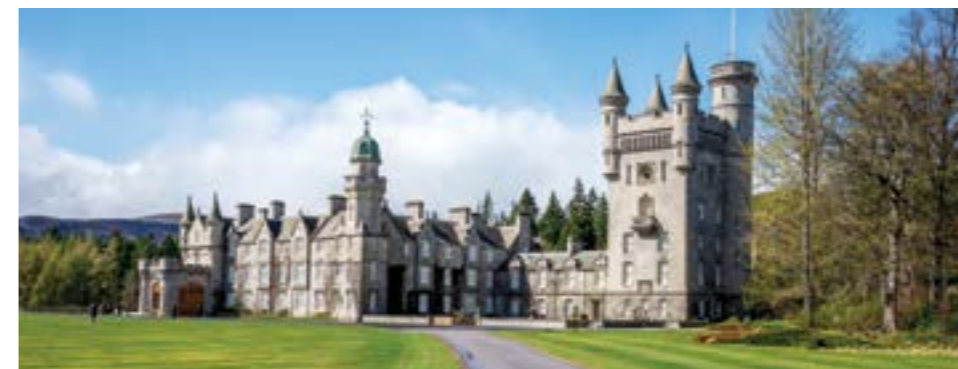
Left: Gilkes is to supply two Francis turbines for a new hydro project on the Balmoral Estate in Scotland
