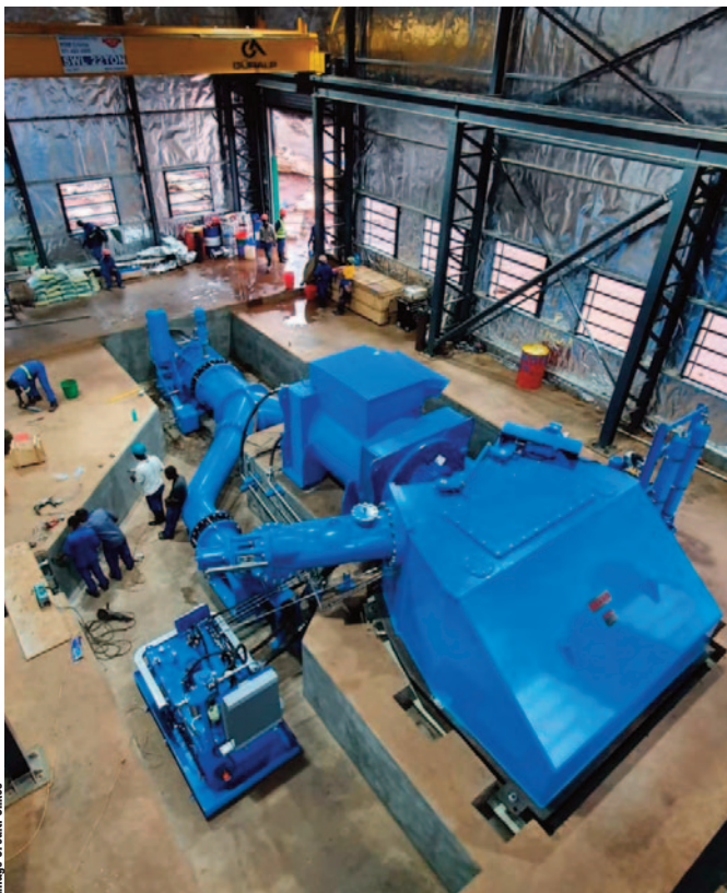
A 3.0MW Turgo turbine has been installed in the Mulosa River project.
