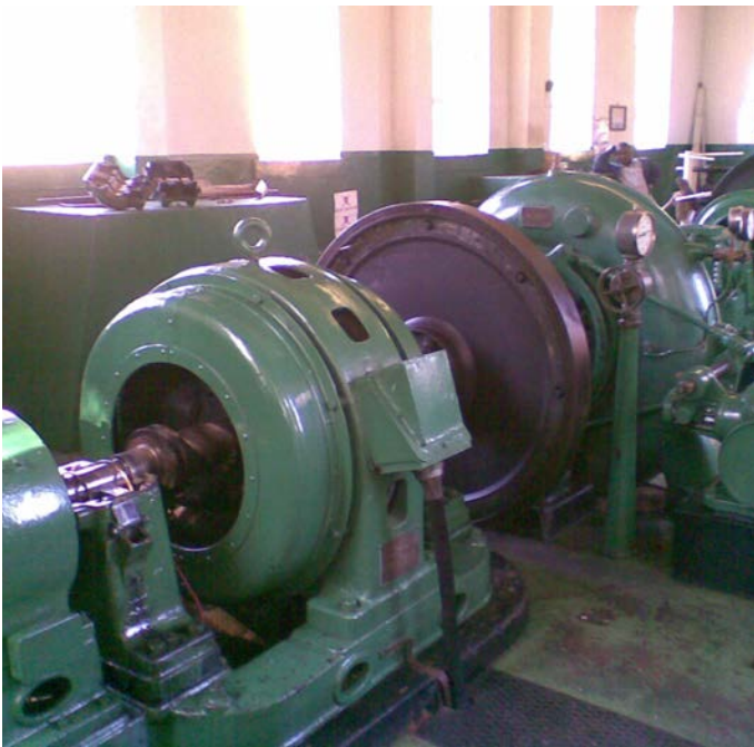
Original Lujeri powerhouse
