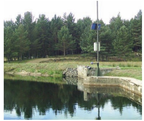
Intake pond head level sensor
