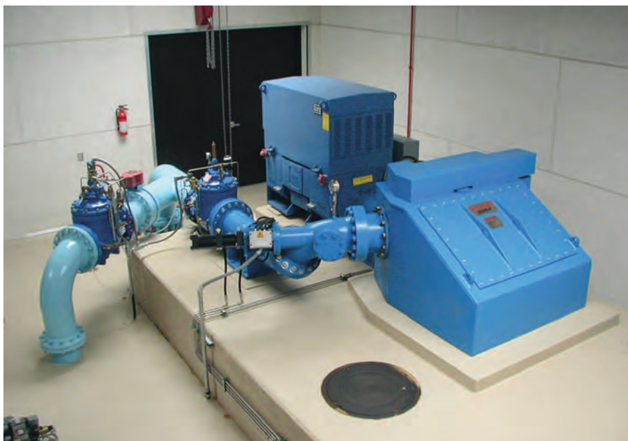
The 12" Compact Turgo unit to be supplied by Gilkes Hydro to AngloGold Ashanti in Mali is very similar to the one pictured
