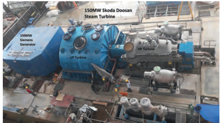
The turbine generator set for Cobre Panama showing the Siemens 150 MW generator and the low pressure and high pressure Skoda Doosan turbine set
