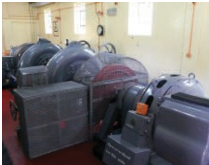
For the five units at the Kerenga hydro plant, governor control initially was achieved through manual operations.
