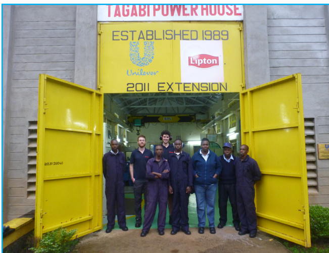
Tagabi Powerhouse after extension
