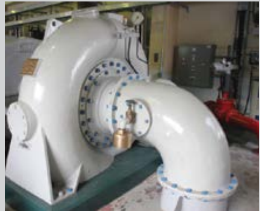
Spiral Case & Discharge Bend upon completion 2013
