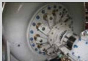
Wicket Gate linkage prior to and post rehabilitation
