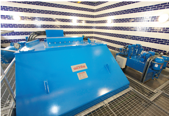
Gilkes turbine installed
