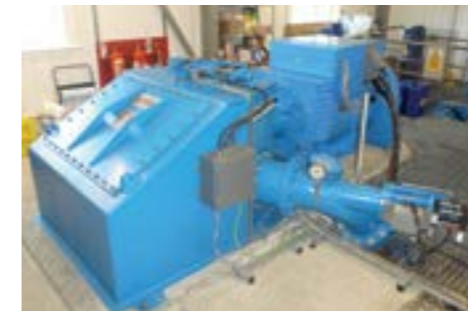
Above: Original 13.5 Twin Jet Turgo installed in 2008
