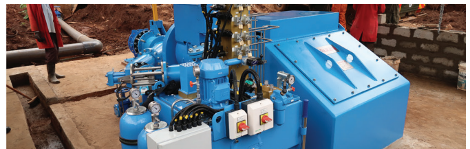
Turbine During Installation
