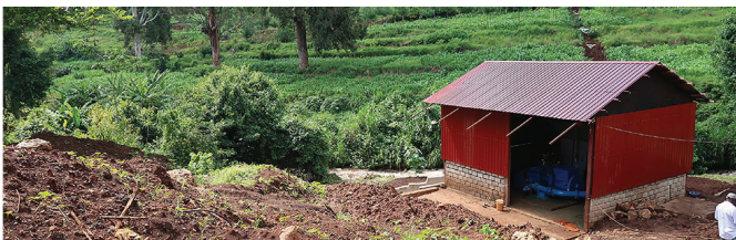
Powerhouse During Assembly
