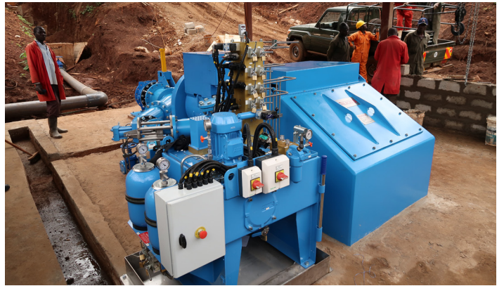
Turbine During Installation
