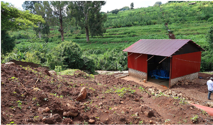
Powerhouse During Assembly
